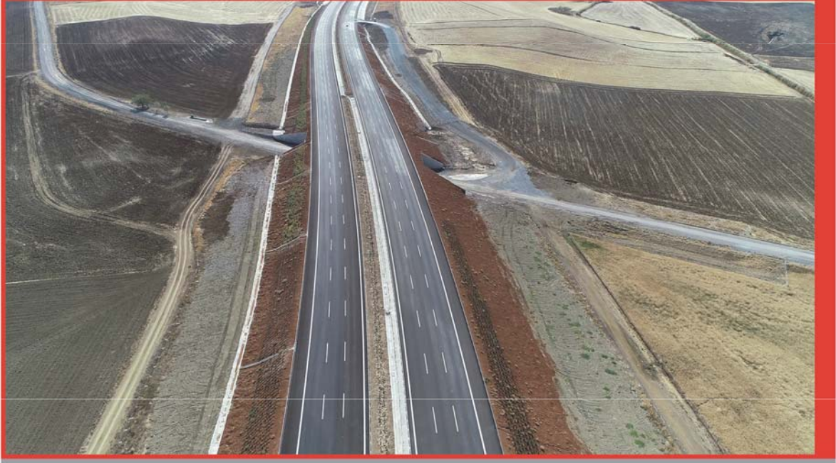
Km: 41+164 Koçyayla-Ahmetçayırı Village Underpass
