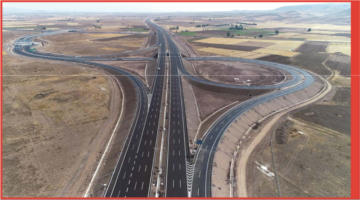
Km: 246+400 Derinkuyu Junction
