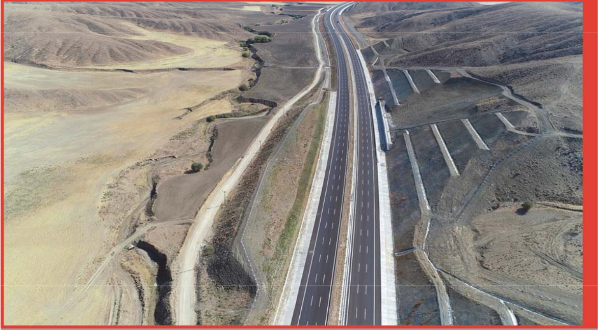
Km: 52+500 Retaining Wall At Cut Section
