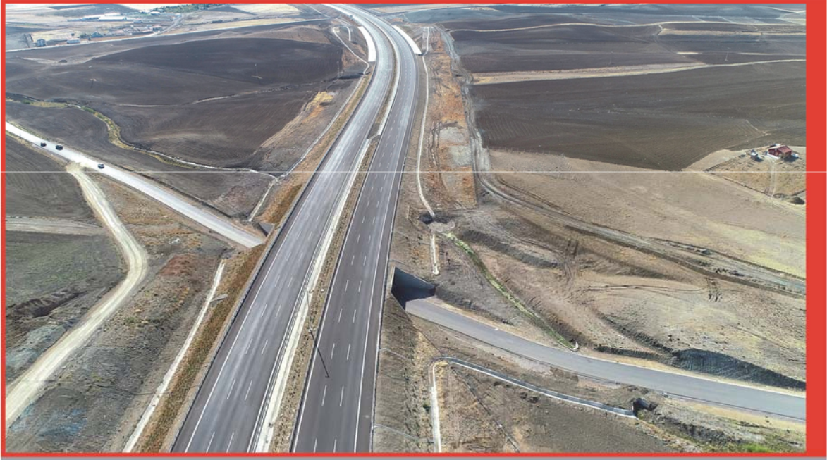
Km: 32+592 Soğulcak Bağı Village Underpass
