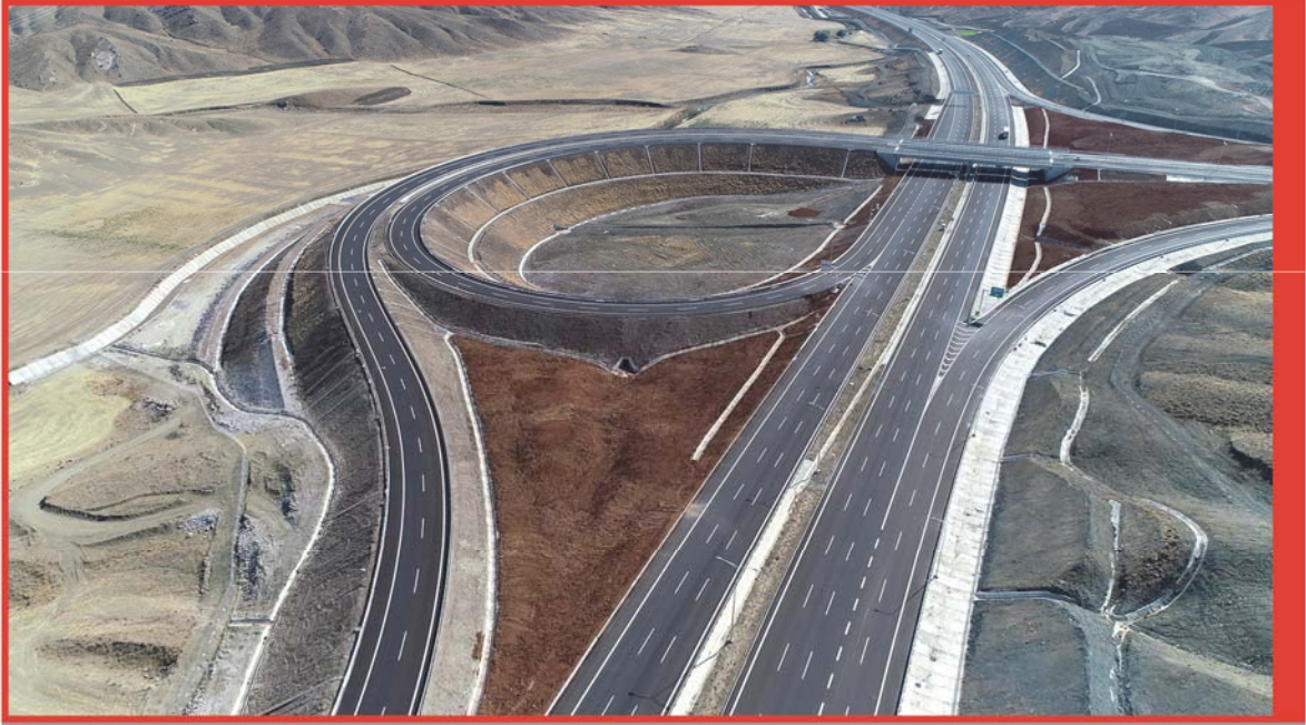
Km: 51+880 Emirler Junction
