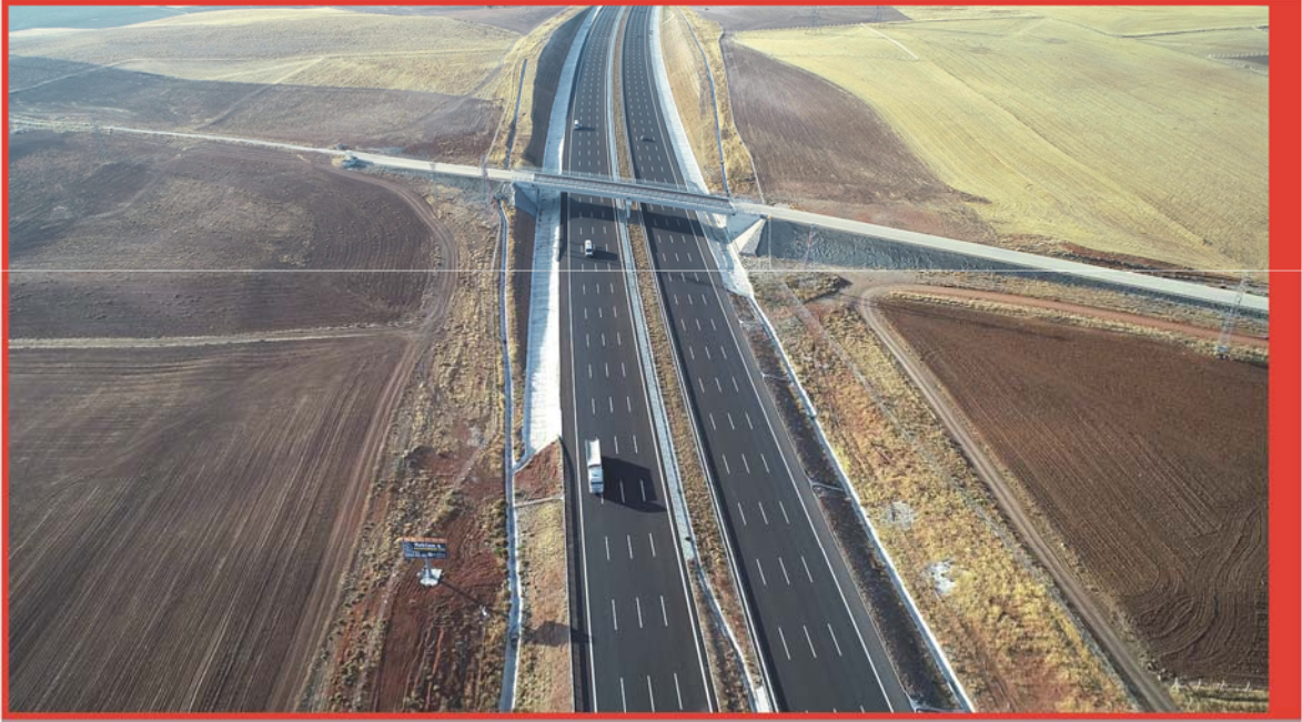
Km: 5+200 Overpass Bridge
