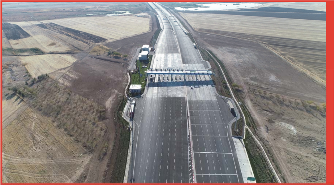
Km: 16+124 Main Toll Plaza
