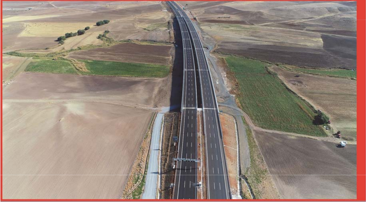
Km: 71+500 Sofular Viaduct
