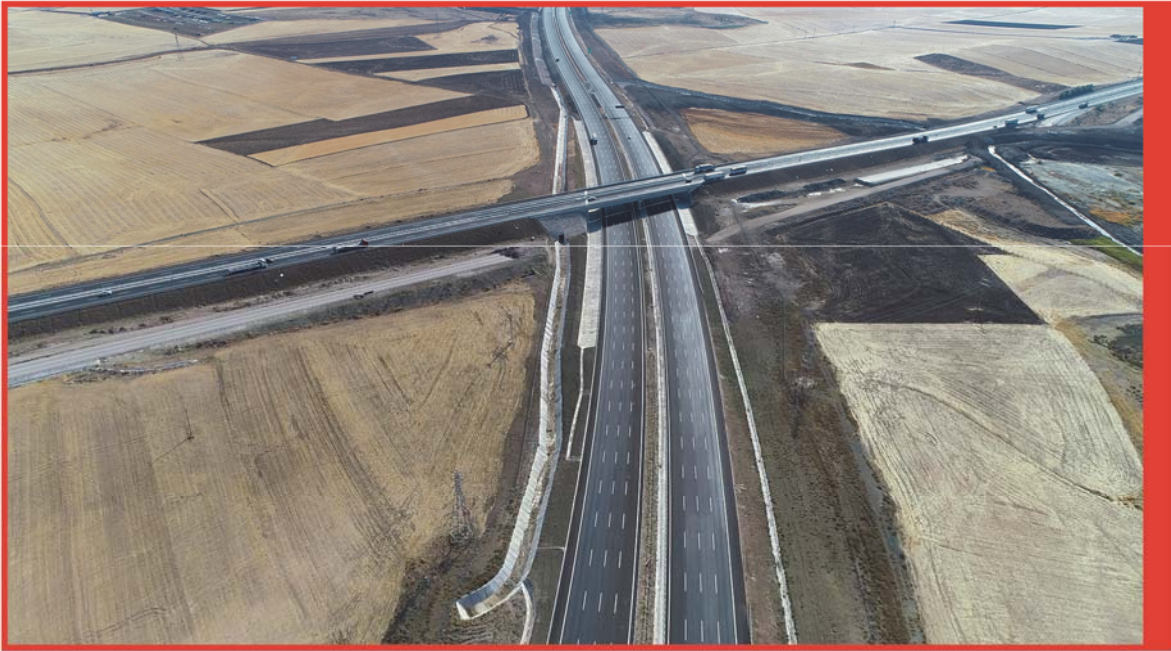
Km: 27+500 Overpass Bridge
