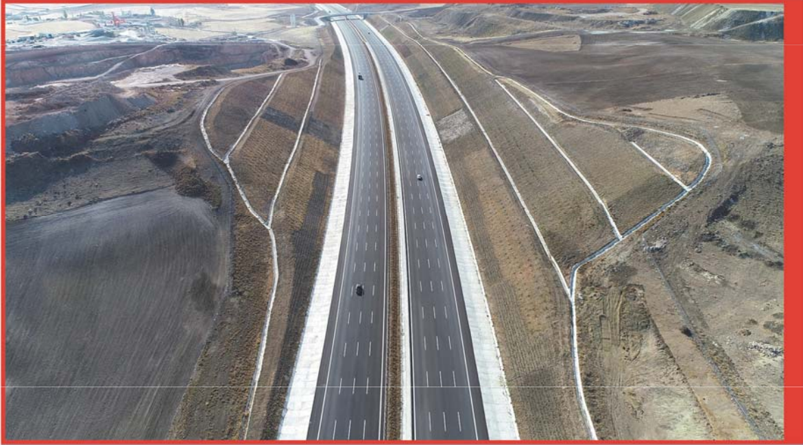
Km: 25+000 Trench Cut
