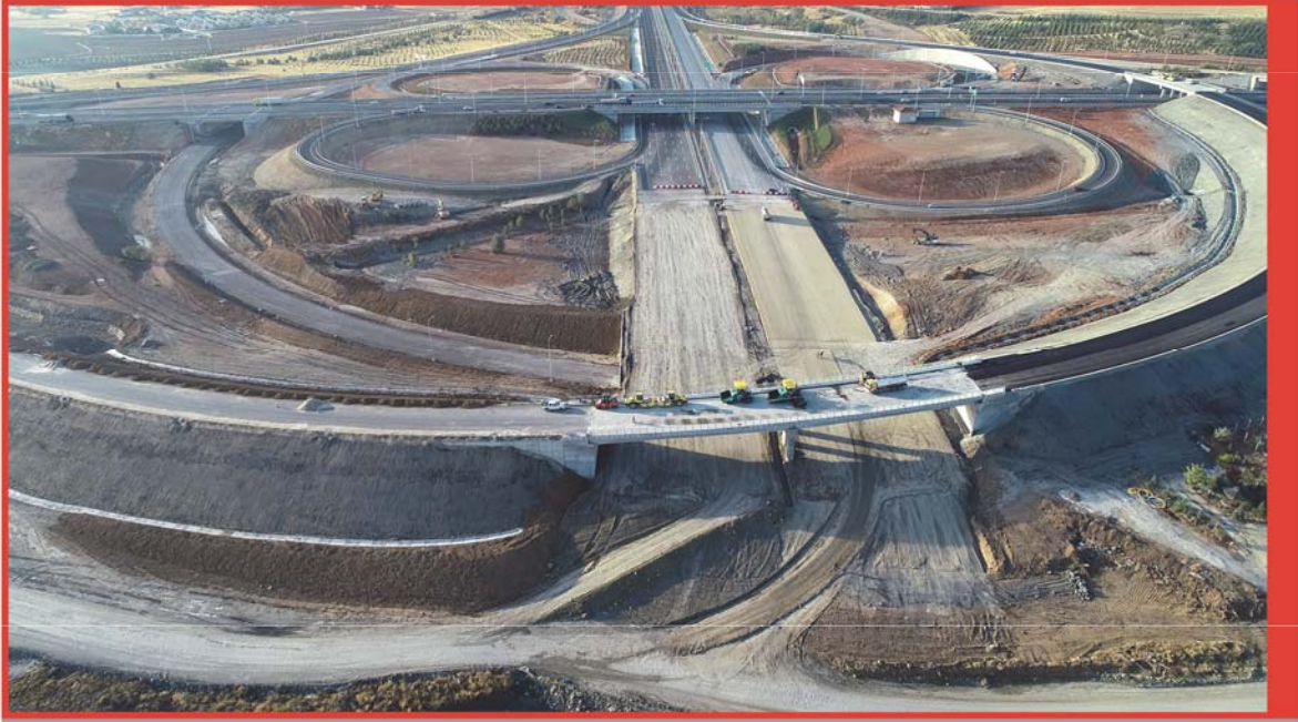
KO Ankara Peripheral Motorway Starting Point Junction
