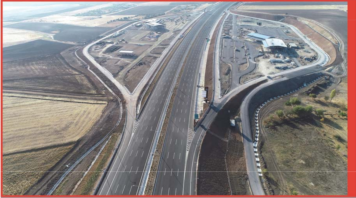
Km: 10+564 Highway Service Facility
