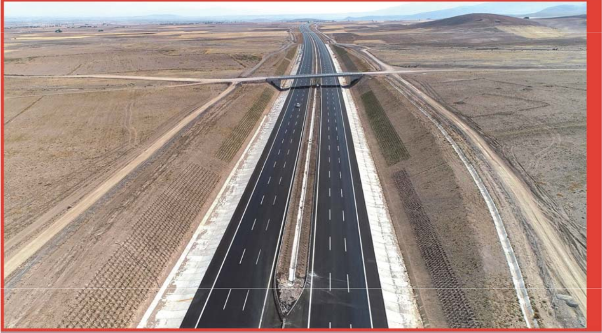
Km: 251+000 Overpass Bridge
